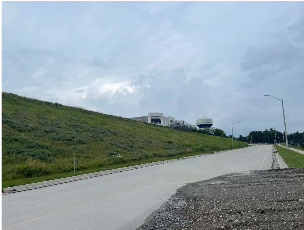
Image 7 – View Northeast of Site looking Southeast along Monarch Park Gate
