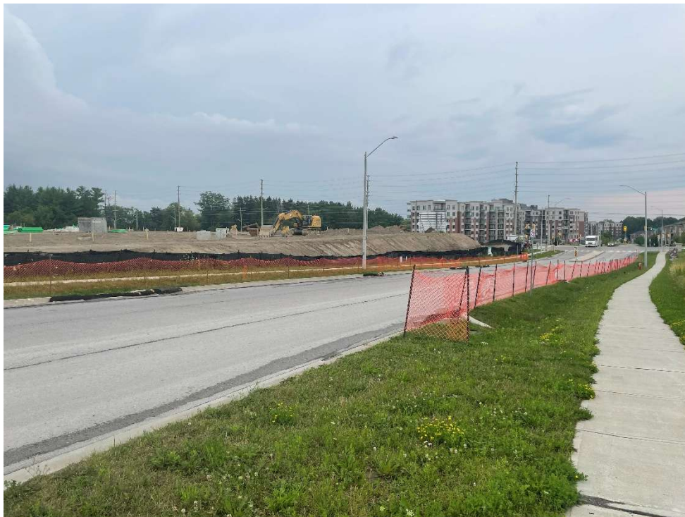
Image 4 – View South of Site looking Southwest towards 25 Addison Hall Cir
