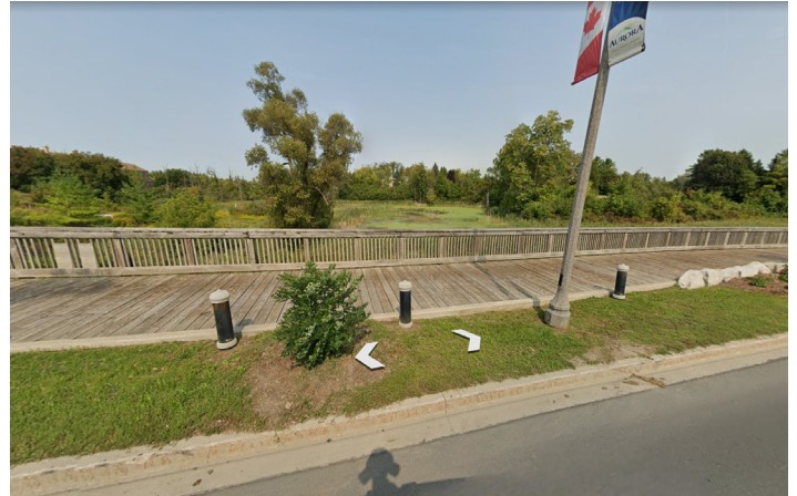
St. John's Sideroad, facing North just East of the subject site
