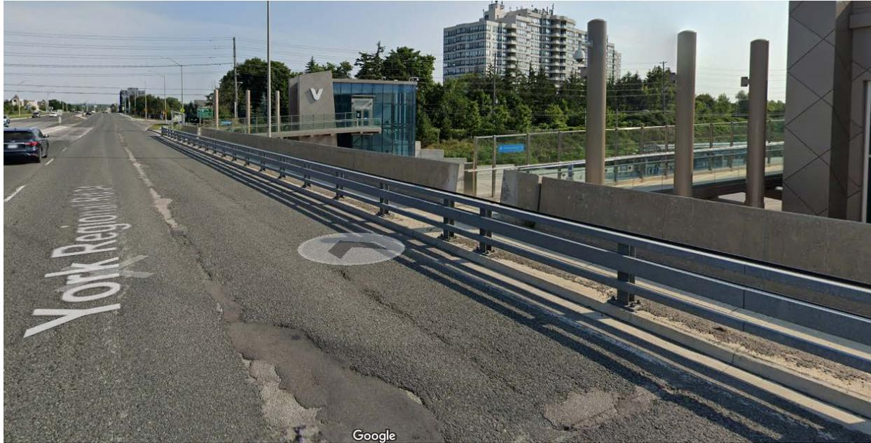
This has led to deterioration of the railings, part of the sidewalk and side support walls and now requires a more significant engineering solution in order to resolve the situation and to mitigate any safety related concerns.
