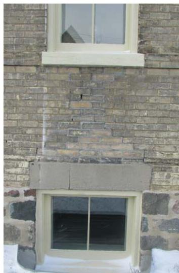
East elevation, showing detail of cracked concrete lintel and cracked and open mortar joints (ERA, 2019).
