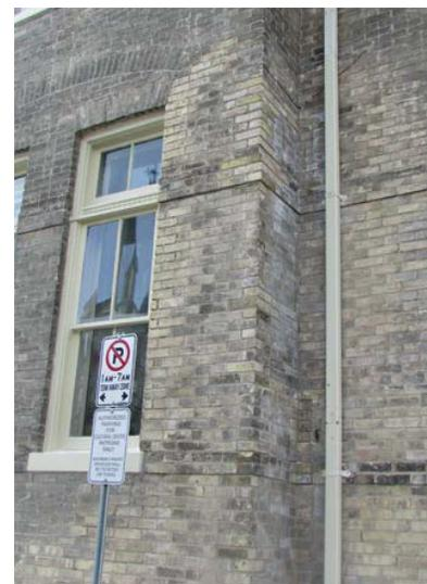
East elevation, showing area of efflorescence (ERA, 2019).
