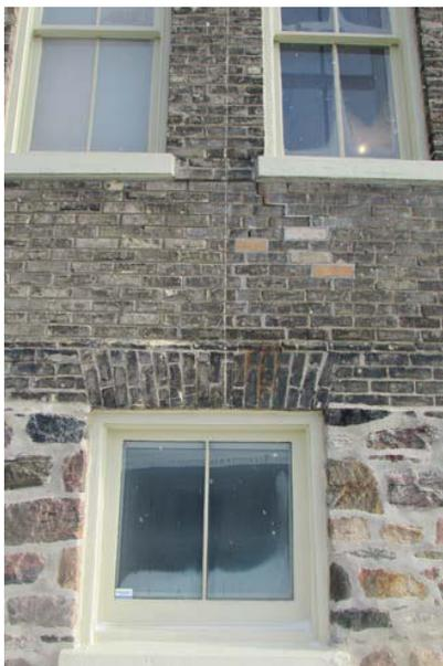
West elevation stone foundation and basement window, showing cracked mortar joints above window (ERA, 2019).
