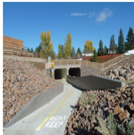
**Figure 3 – Twinned Culvert/Pedestrian and Cyclist Crossing**
