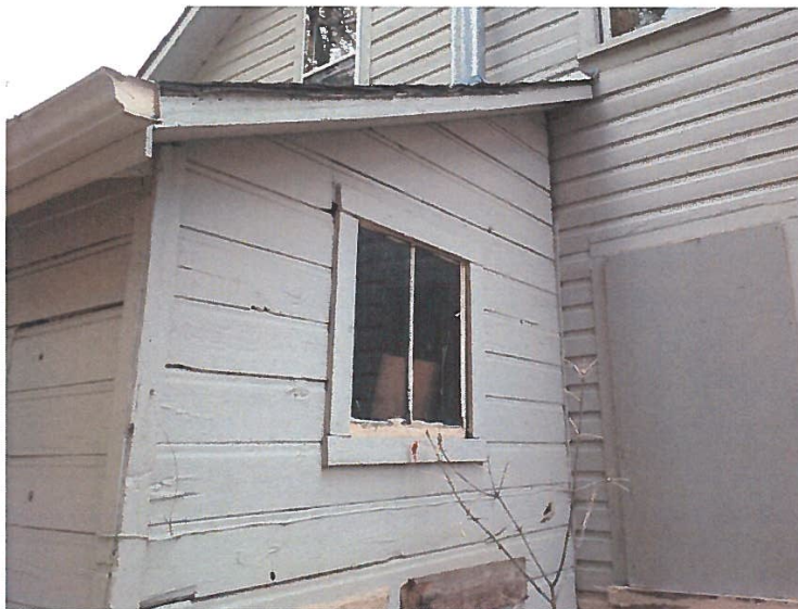
Photo of Accessory Structure (Mudroom) looking southeast
