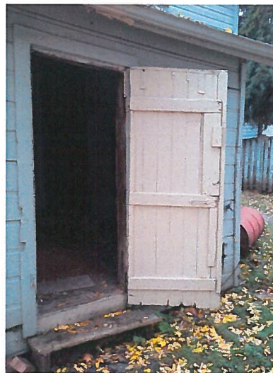
Photo of Accessory Structure (Mudroom) Door
