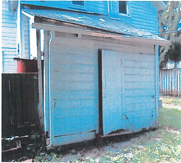
Scanned Photo of Accessory Structure (Mudroom) looking South
