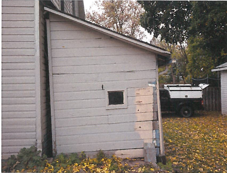
Photo of Accessory Structure (Mudroom) looking West
