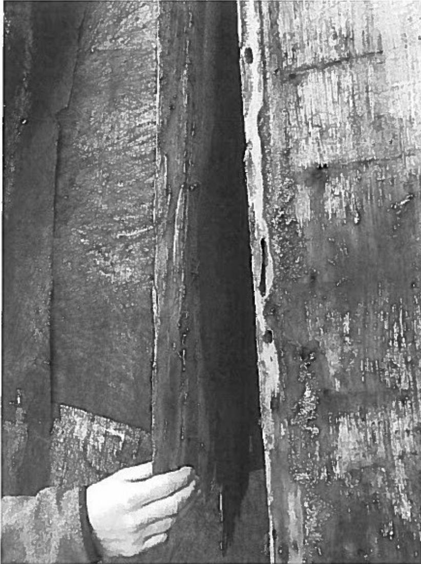
**Photo 6. Evidence of carpenter ant activity in the walls above the sill beam (wood shavings and ant galleries).**
