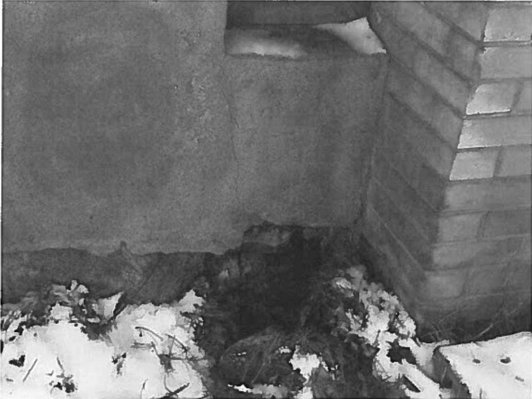
Photo 4. Loose foundation stones along the west side.
