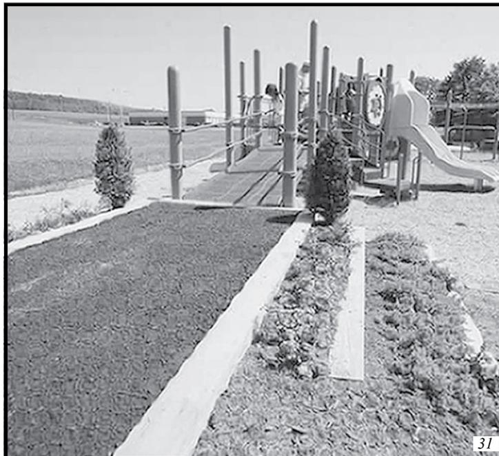
*To accommodate a height change along the perimeter of a playspace – like these rubber safety tiles placed on an asphalt surface – an allowable 1:12 slope is utilized for the transition at the boundary of the playspace.*
