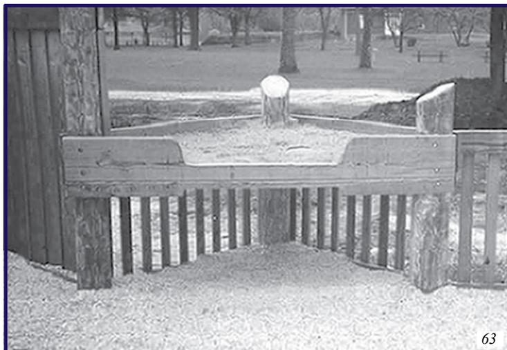
*The edge of this elevated sand table has been designed to provide access by providing a generous opening. The tops of rims, curbs, or other obstructions that would prevent access to a table surface should be 787 mm (31.0 in) maximum in height.*
