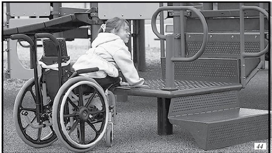
Where a transfer system is provided, a combination of transfer platforms and transfer steps provide a continuous accessible route to elevated play components. A transfer system provides individuals the space necessary to physically transfer up or down in a composite play structure. Where provided, a 610 mm (24 in) minimum width is necessary for individuals moving around a structure.
