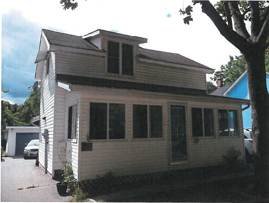
Existing front façade, looking west
