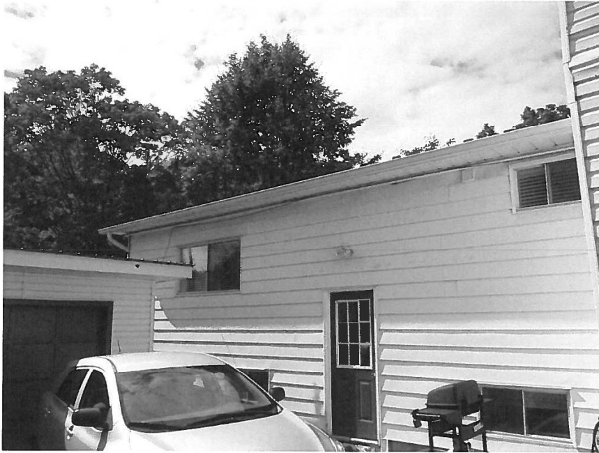
Existing rear addition
