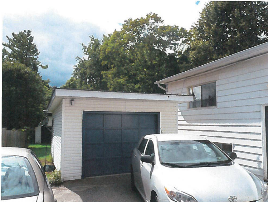
Existing Garage, proposed to be demolished
