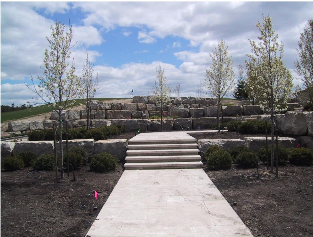
**Examples of Armour Stone Retaining Walls**
