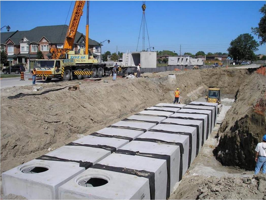
Subsurface Stormwater Storage Facility
