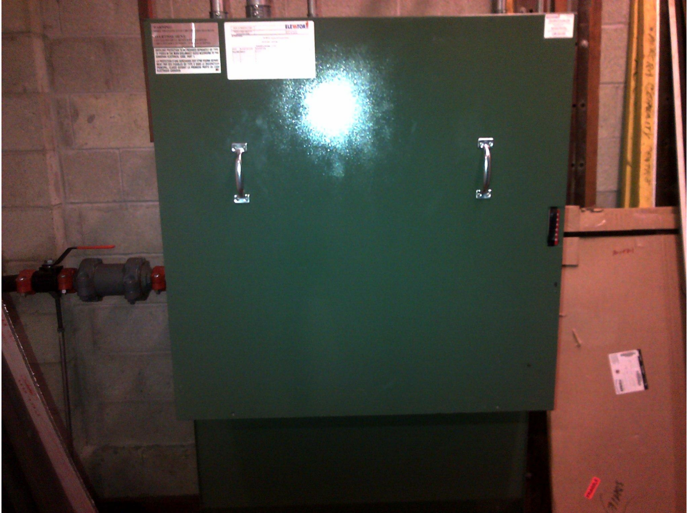
C:\Users\Phillip Galin\Pictures\ACC Elevator 3.jpg
