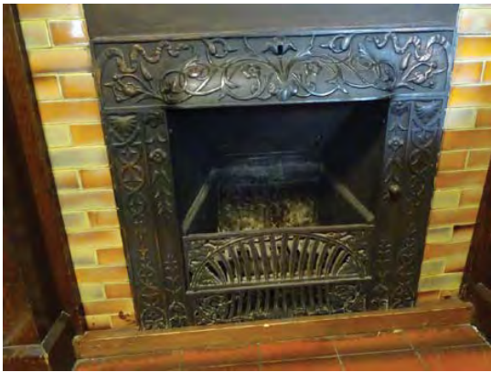
Above: Ornate metal firebox with glazed tile surround and clay tile hearth
