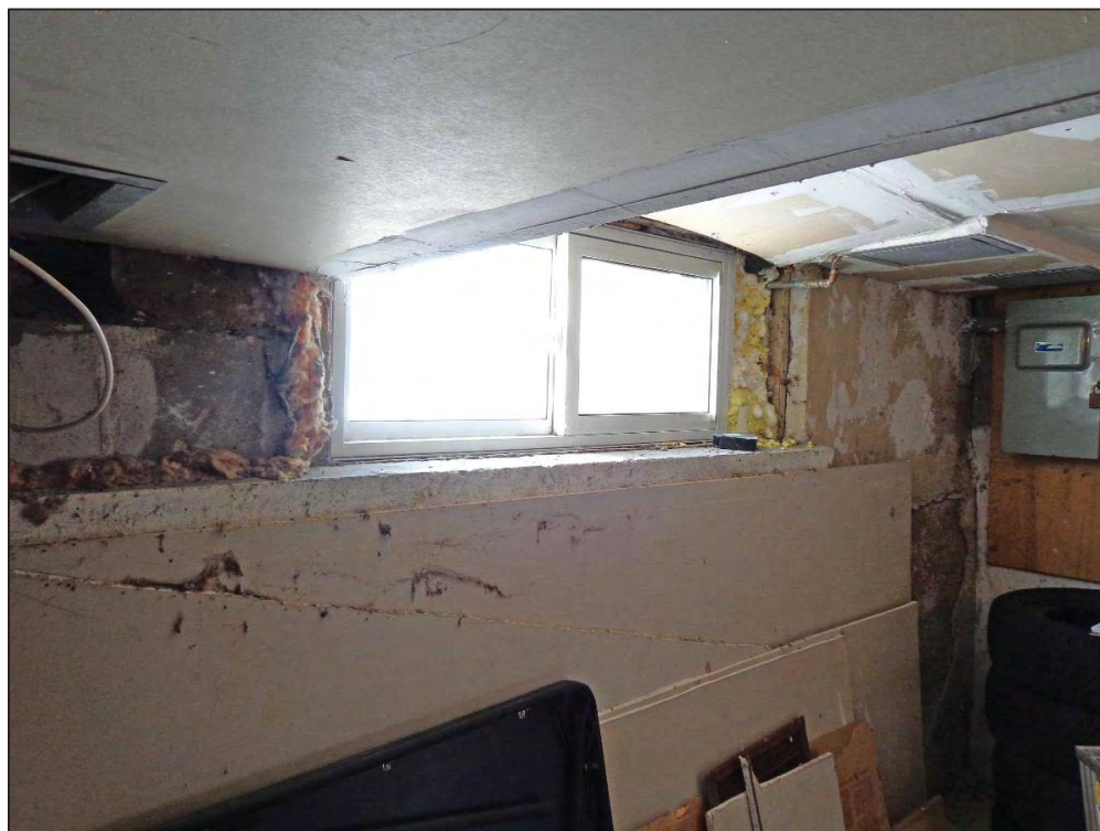
6. Room 3 – South Wall.
