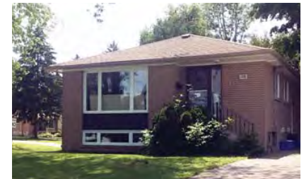
Example of a slightly recessed entrance feature covered by the main roof
