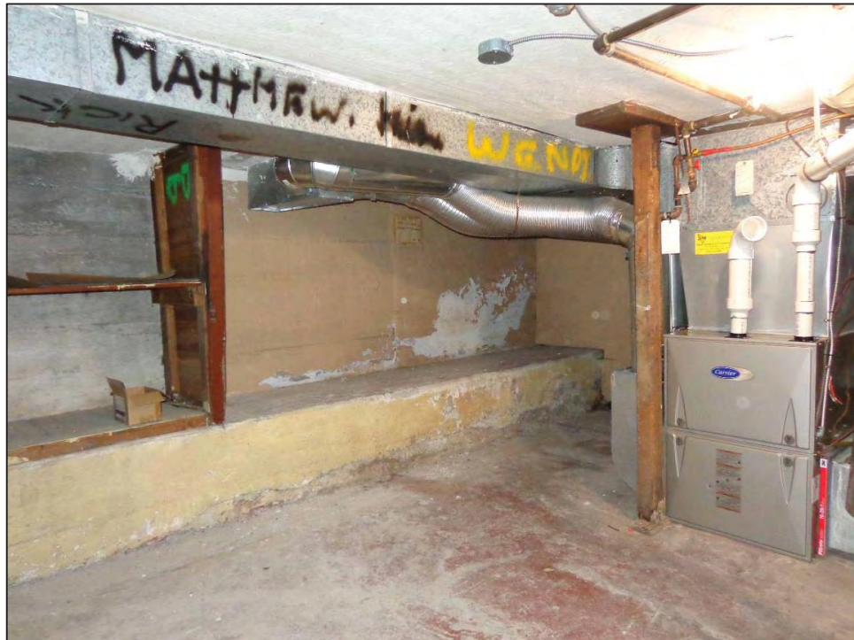
8. Room 3 – Furnace Room – South and East Walls.
