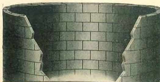
Showing Curbing Built In
