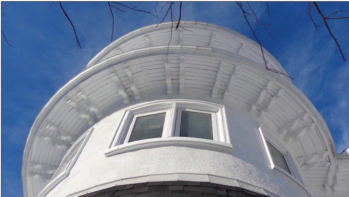
Eave Detail, Corner Tower, East Elevation.
