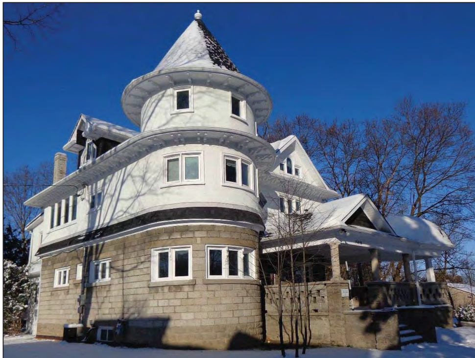
South and East Elevations
