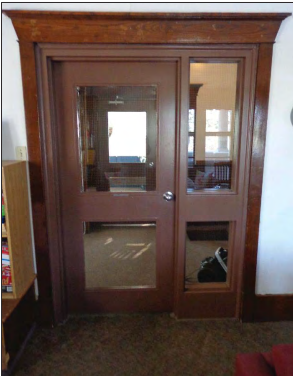
19. Room 5 – Door – East Wall, South end.
