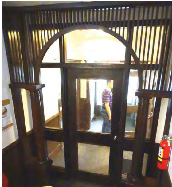
Beside: Wood screen between entry and stairwell
