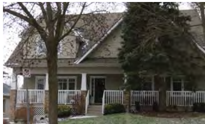
Wood clapboard as primary material with stone used as accent and metallic railings complementing the dwelling's architecture
