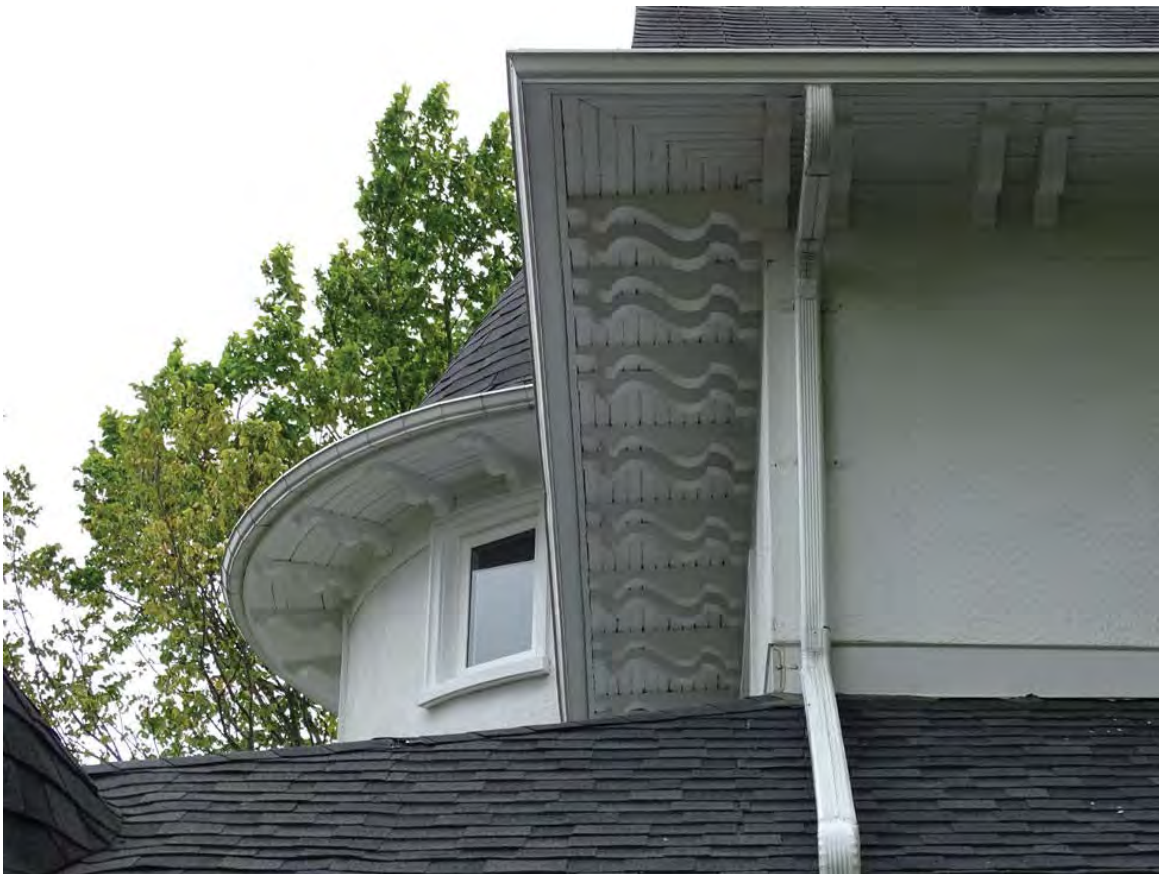
Tongue and Groove Wood Soffit with Paired Brackets
