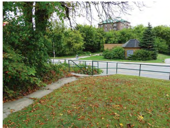
Pavers Leading to South Stairs to Yonge Street
