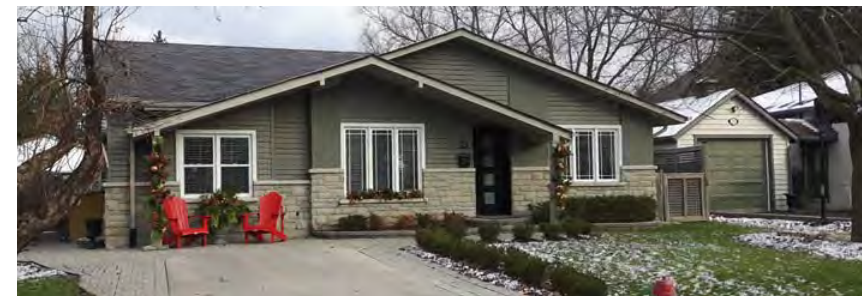
Entrance at grade, covered by main dwelling’s roof and connected to the lot’s access
