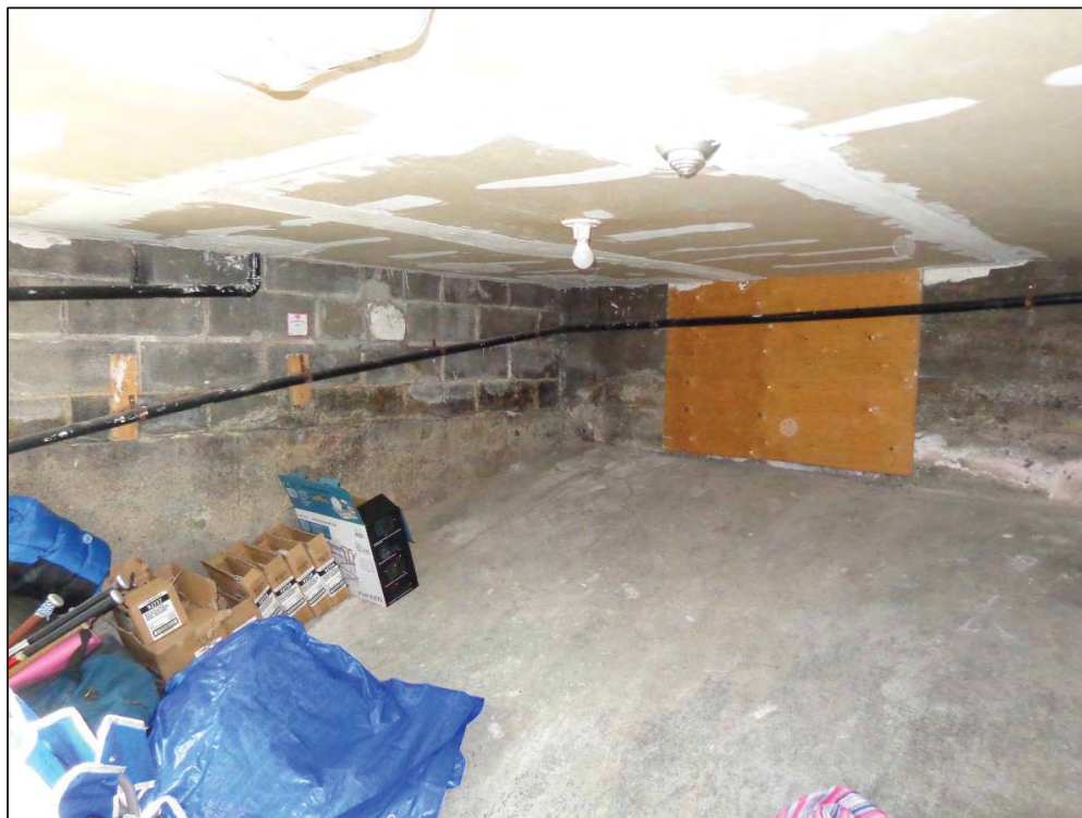
4. Room 2 - South & West Walls.
