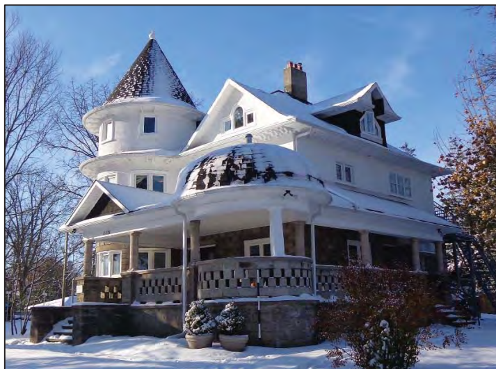
Figure 5.1 House at 15074 Yonge Street, East and North Elevations, 2019
