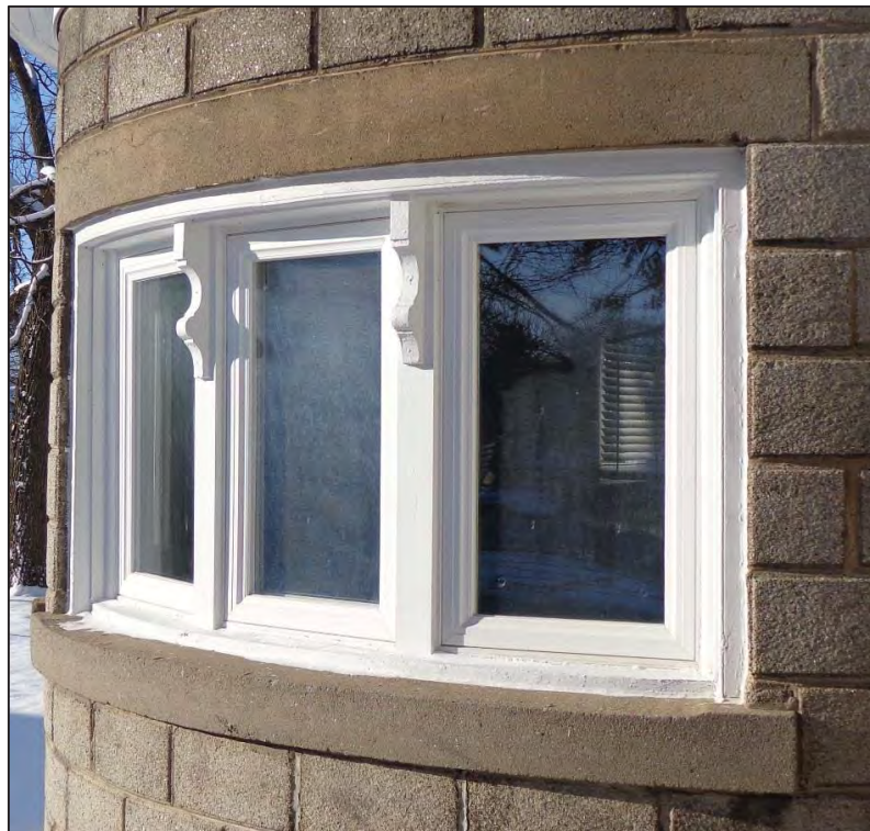
Ground Floor Tower Window Detail, East Elevation.
