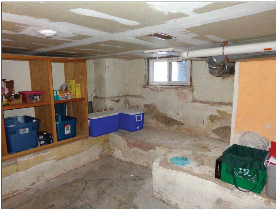
2. Room 1 – West and North Walls.
