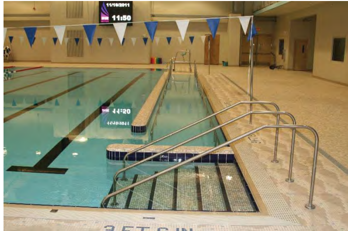
Permanent Built in Ramp and Stairs
