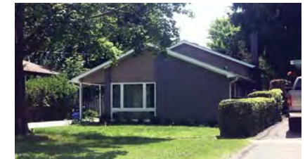
Shallow pitched roof lines complement simple building geometry
