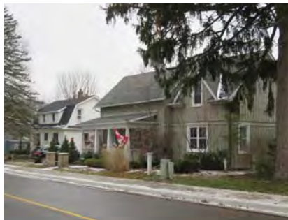
Siding, as well as brick, are common materials
