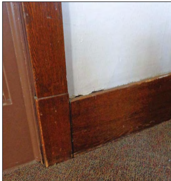
20. Room 5 – Door Casing & Baseboard Detail.
