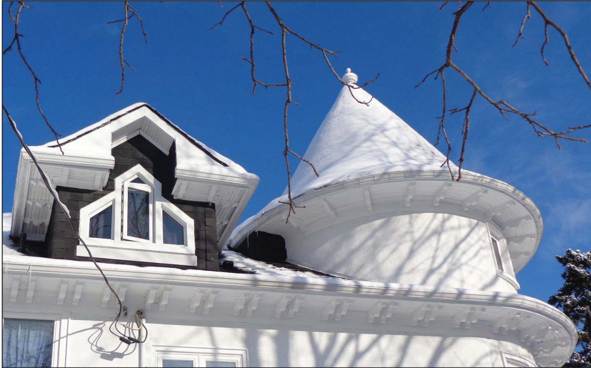
Dormer and Corner Tower, South Elevation.
