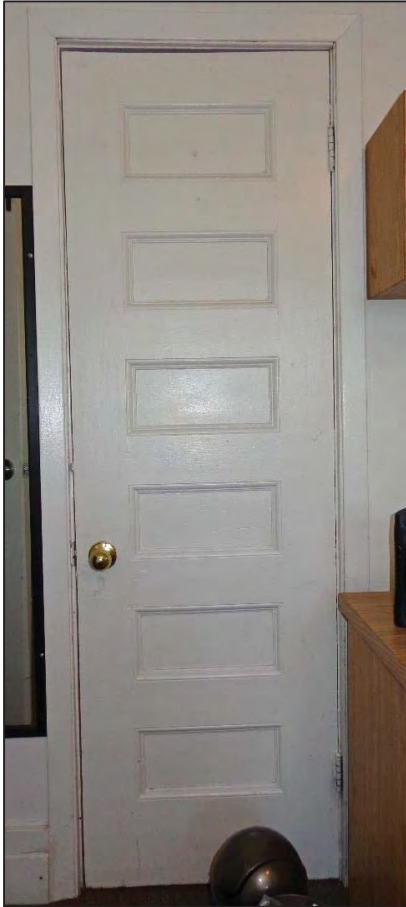
10. Room 2 – Closet Door.
