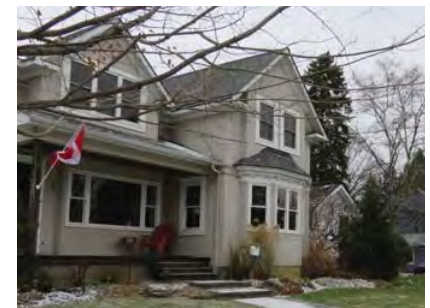
Articulated elevation with changes in plane and pitched roof lines
