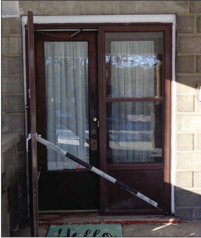
Front Door, East Elevation
