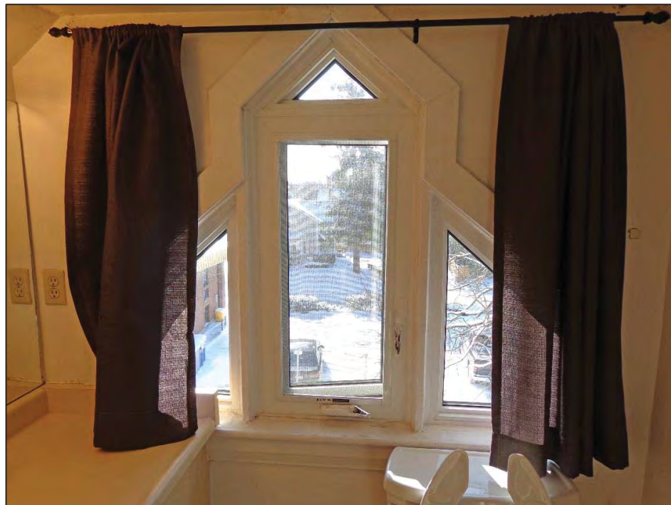
10. Bathroom – Window on south wall.
