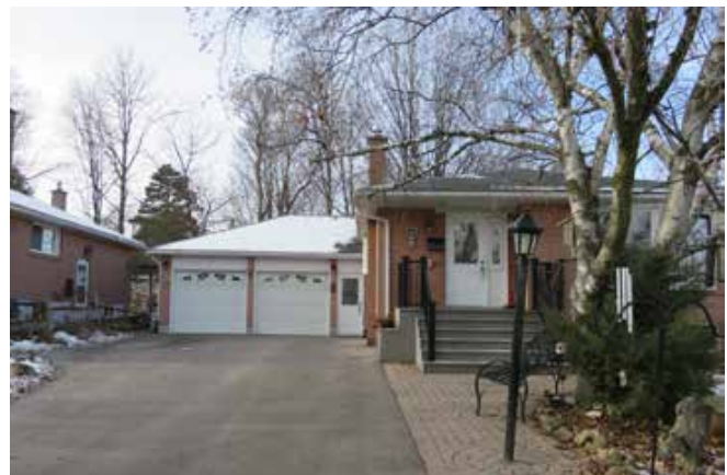
Example of a modest street oriented front entrance.
