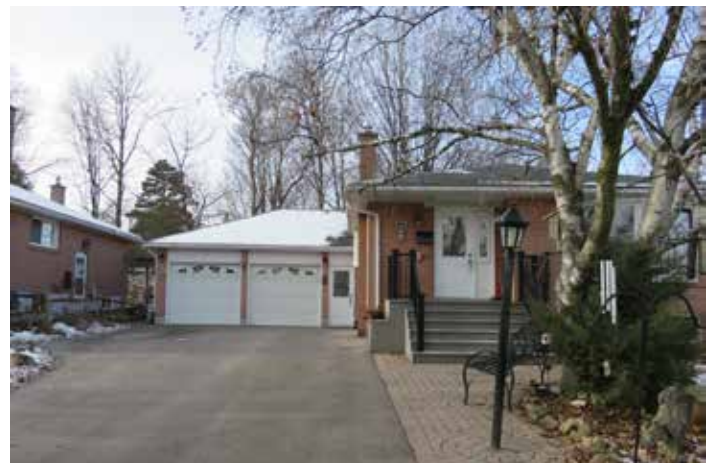
Example of a modest street oriented front entrance.
