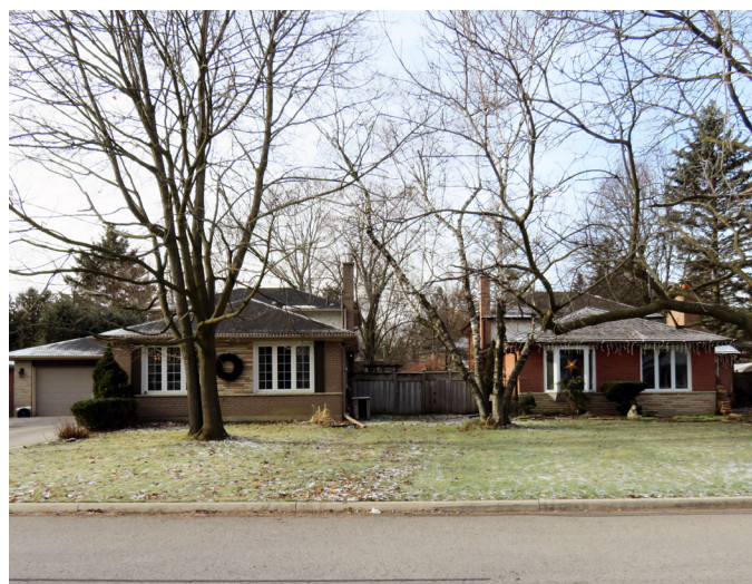
Mature trees and extensive grassed areas dominate front yards
