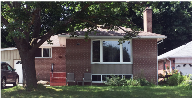
A variety of wood clapboard and brick are extensively used as primary materials
