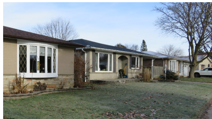
A consistent building height of 1.5 storeys frames the streetscape
