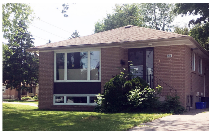
Example of a slightly recessed entrance feature covered by the main roof
