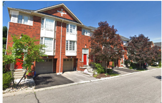
Looking northwest towards townhouse buildings along Mosaics Avenue
