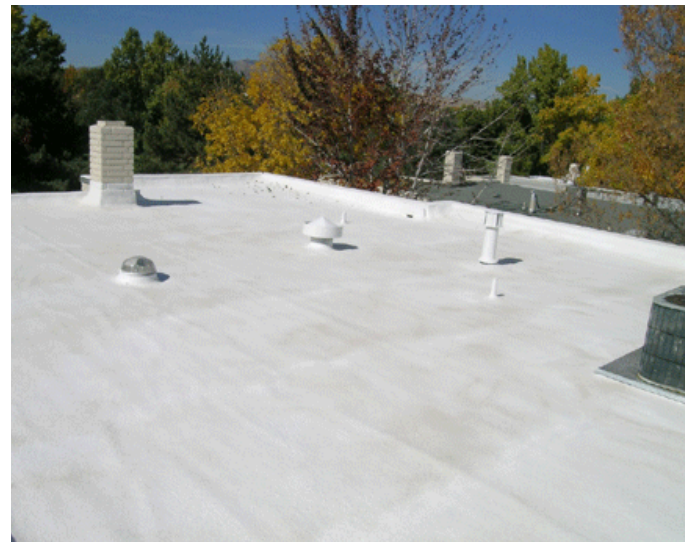
Figure 13.4 Example of a high albedo roof finishing to reduce urban heat island effect.
