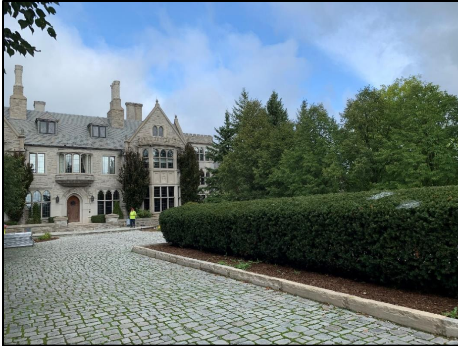
Photograph 7. Existing Dwelling and Future School Structure (September 10, 2020)
