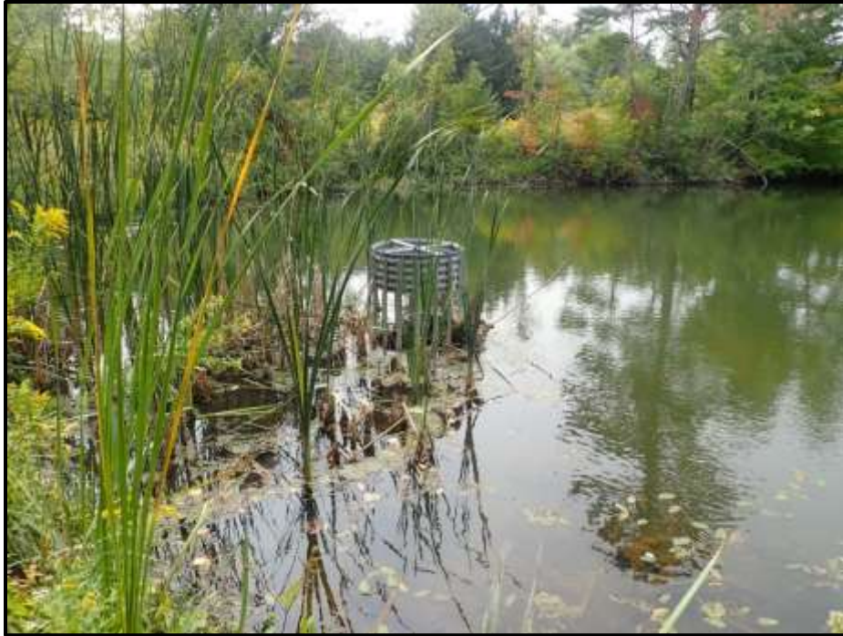
Photograph 3. Tannery Creek West Tributary – Online pond Drainpipe (September 16, 2020)
