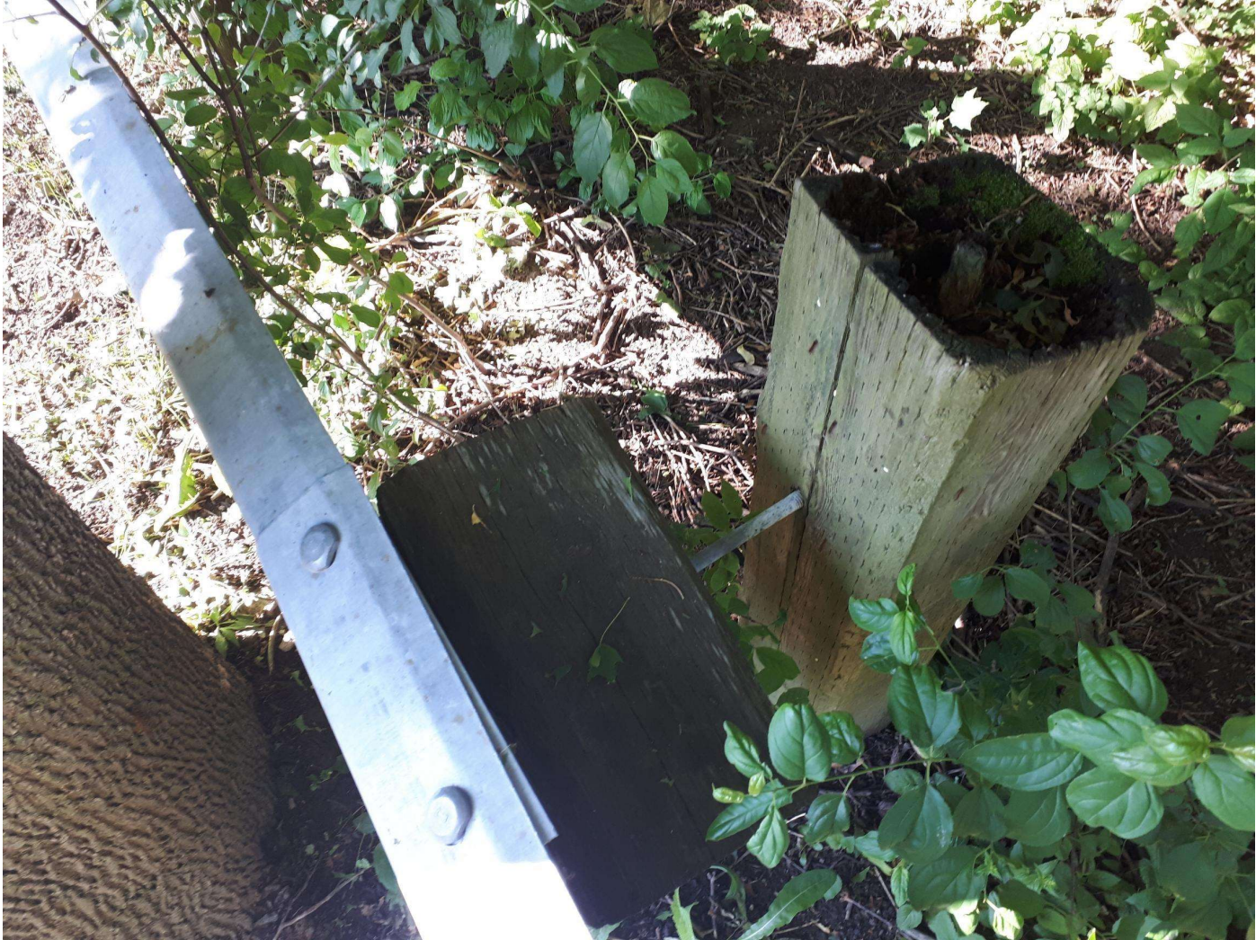
C:\Users\LColangelo\Pictures\Marksbury Court Guiderail\Pic 3.jpg
