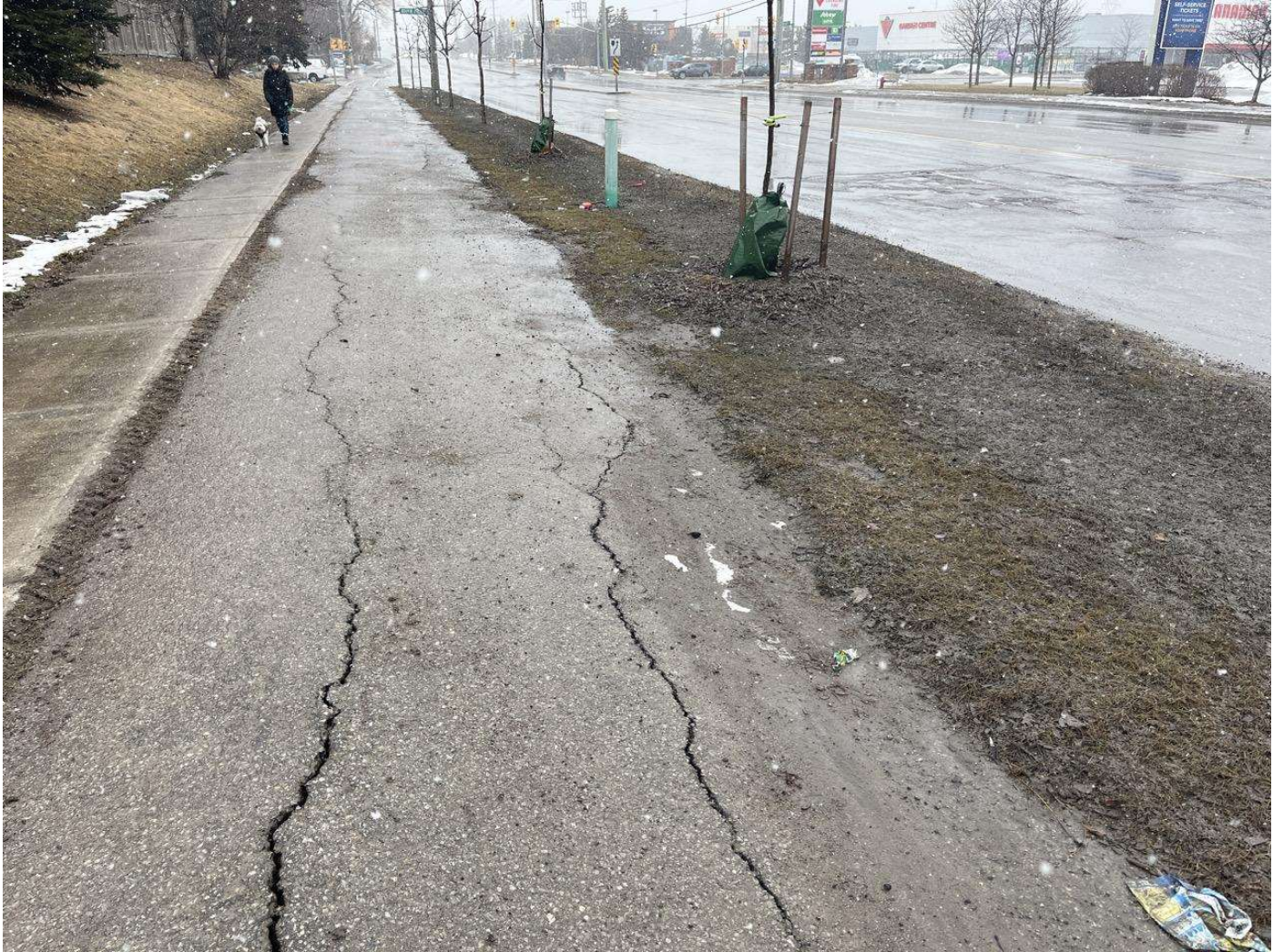
C:\Users\LColangelo\Pictures\Multi-Use Path on Bayview Avenue\Photo 9.jpg
