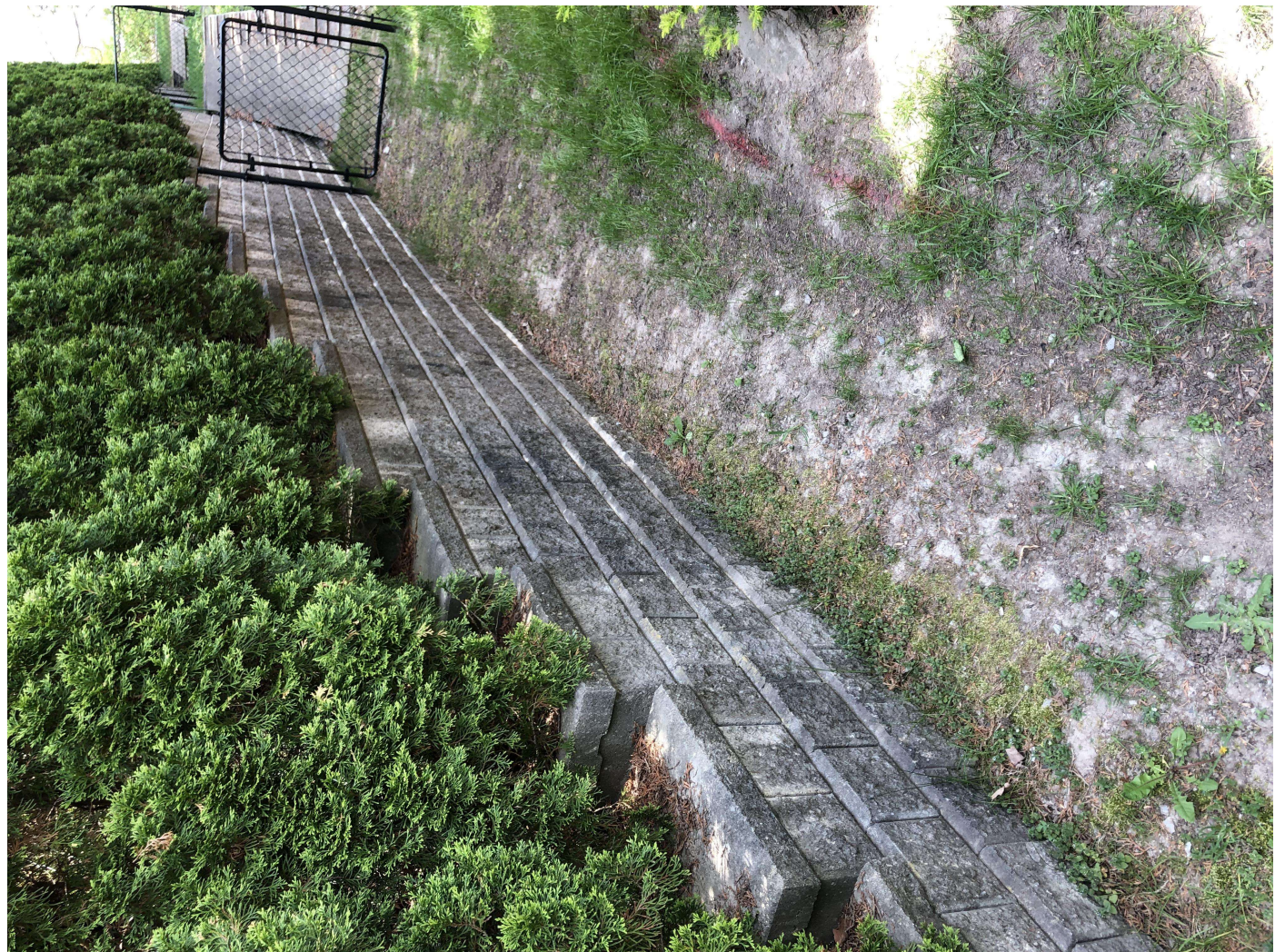
C:\Users\LColangelo\Pictures\Retaining Walls\IMG_5502 (002).JPG
