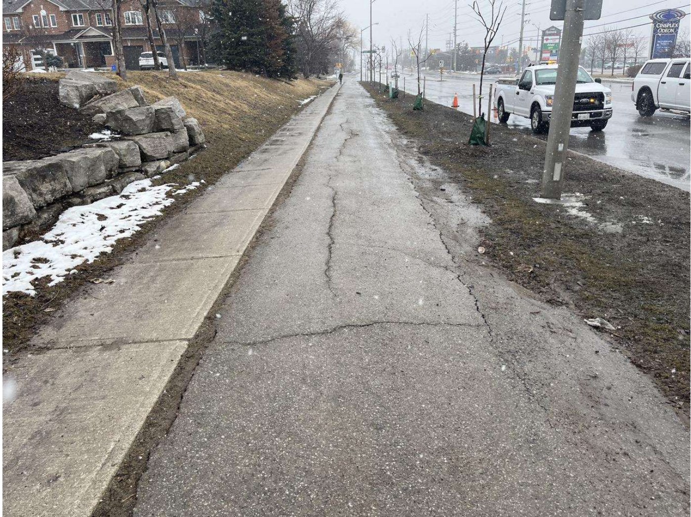
C:\Users\LColangelo\Pictures\Multi-Use Path on Bayview Avenue\Photo 7.jpg
