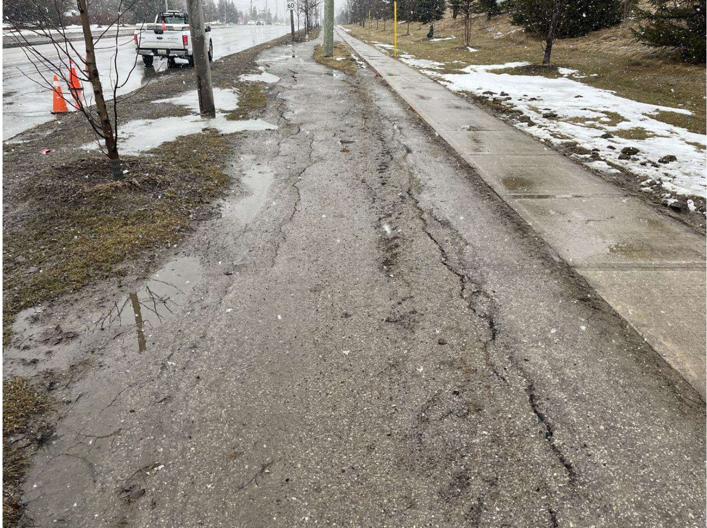
C:\Users\LColangelo\Pictures\Multi-Use Path on Bayview Avenue\Photo 5.jpg
